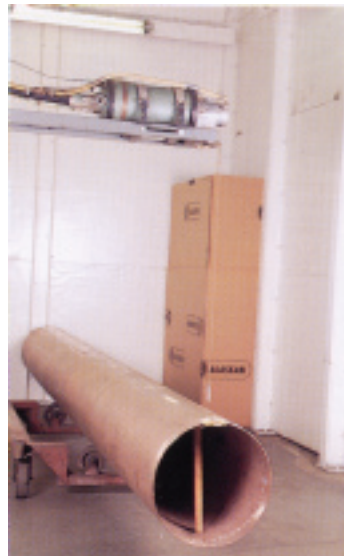
Radiographic inspection checks the integrity of welds.
