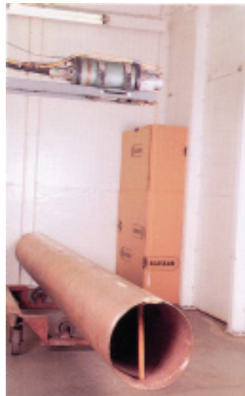
Radiographic inspection checks the integrity of welds.
